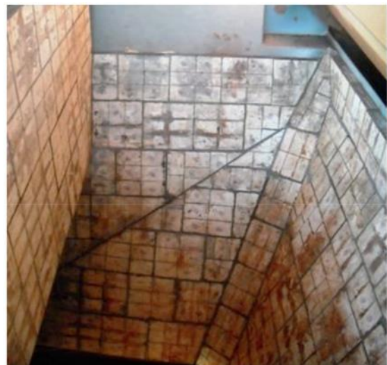
CorroTile™ liners installed in a reclaimer chute.
