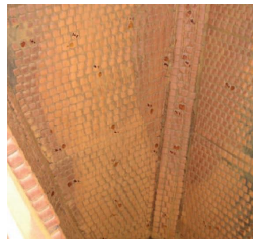
CorroCube™ liners installed in an iron ore apron feeder chute.
