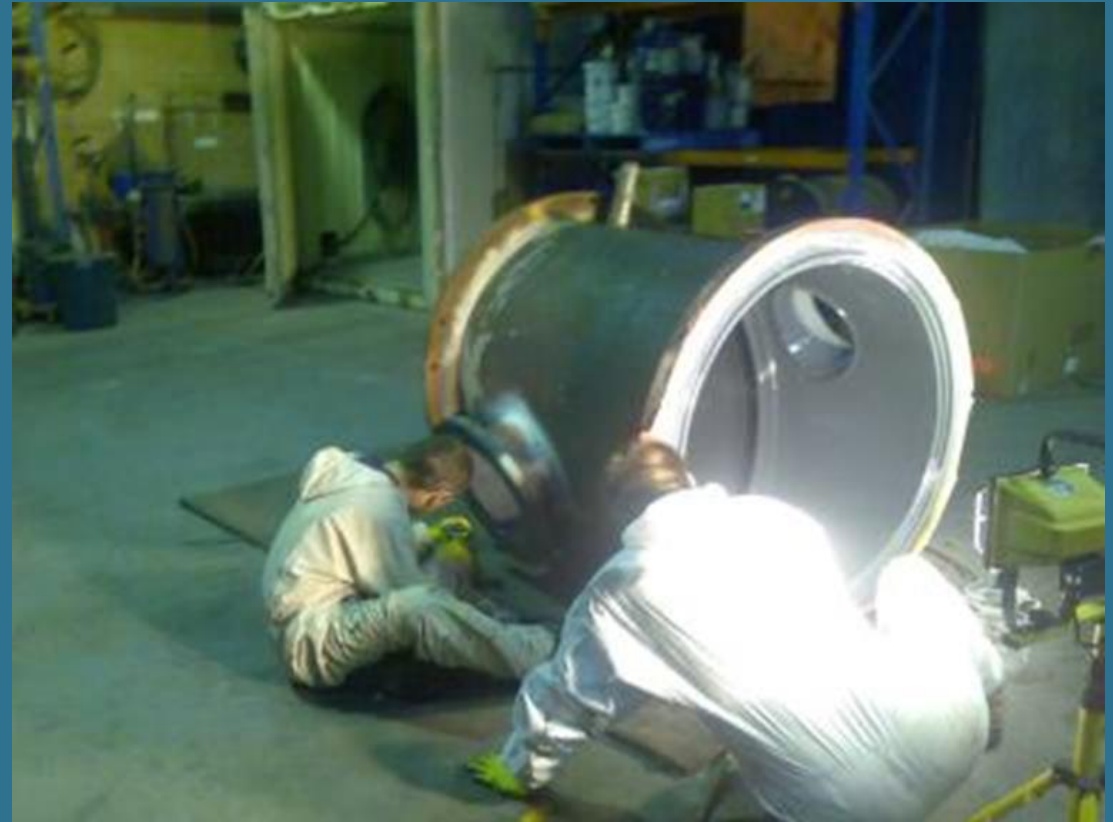
Stripe coating welds
