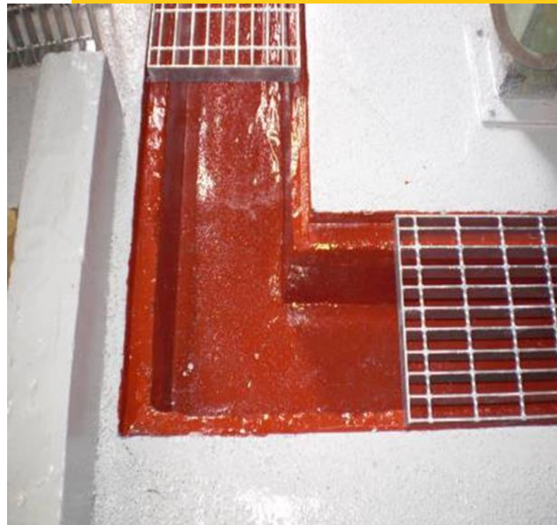
Final Coat ARC CS2 and ARC CS4
