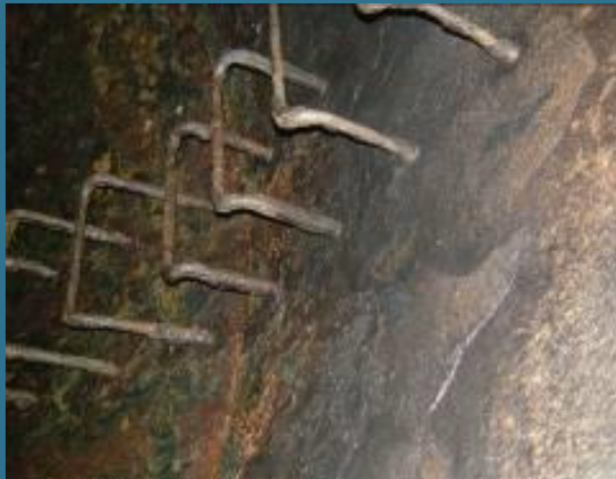
Condition prior to re-grading
