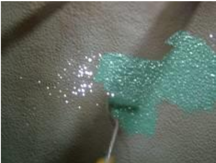
Prime coating with ARC S2 Green
