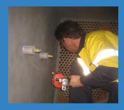
After welding, all surfaces to be Chesterton® ARC coated were abrasive blasted to SA  $2\frac{1}{2}$ , with an angular profile between 75-125 microns. The welders could not reach behind the titanium plate, so Chesterton® ARC 858 was "injected" into the cavities and around the edging of the tube sheets.
