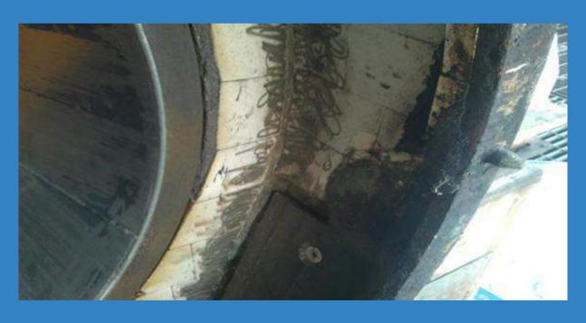
The area was prepared using a grinding disc and a needle gun.
