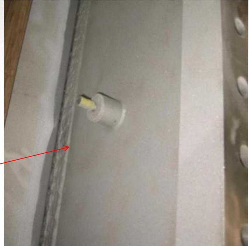
Specialised welders were brought in to close the holes and build up as much metal on the carbon steel as possible.
