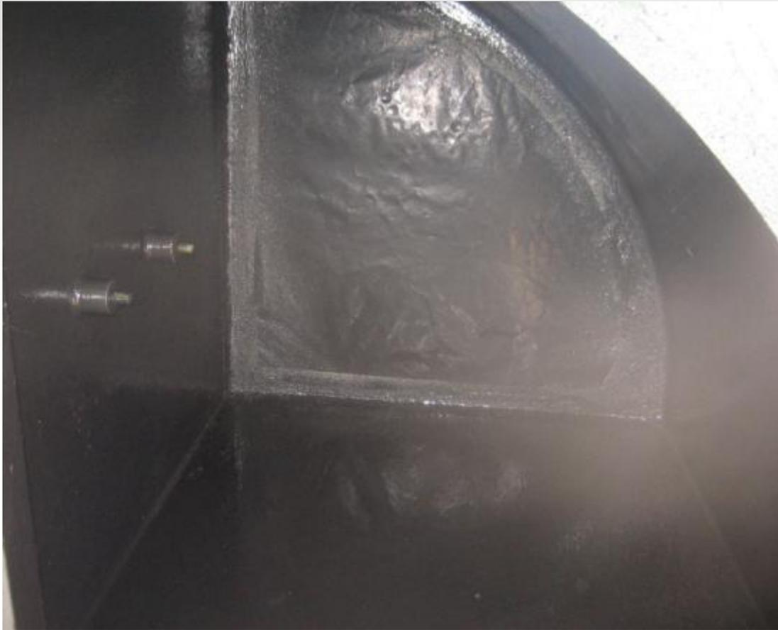
Finally, 2 x 350 micron coats of ARC 855 HT were 'sprayed on' to ensure total corrosion protection from the sea water, which operated in temperatures up to 120<sup>0</sup> C.
