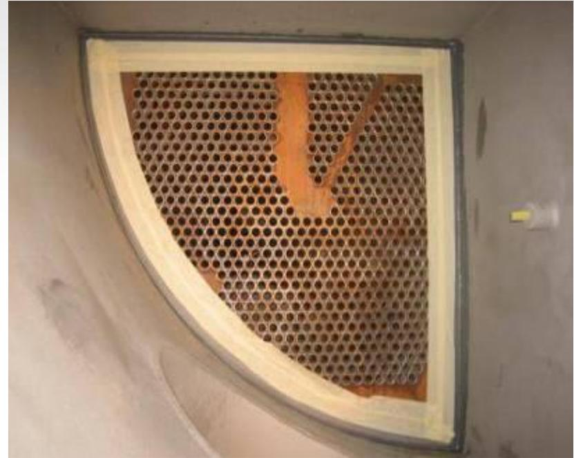
After welding, all surfaces to be ARC coated were abrasive blasted to SA 2½, with an angular profile between 75 – 125 microns. The welders could not reach behind the titanium plate, so ARC 858 was “injected” into the cavities and around the edging of the tube sheets.
