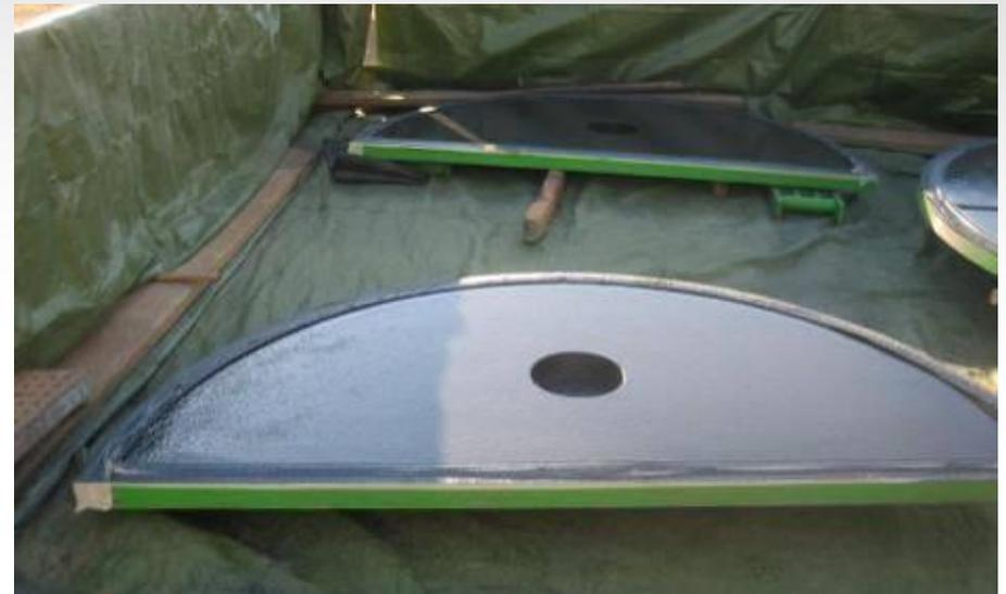
Finally, the end caps were also coated with 2 coats of ARC 855 HT. A four year warranty was given to insure them against product and application failure.
