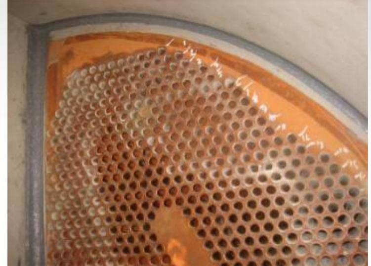
To ensure the corners were totally sealed, a 20 mm edging of ARC BX2 was applied over the ARC 858.
