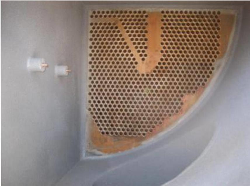
The titanium tube face had shown no corrosion, so no coating was necessary.
